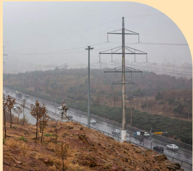
132 kV transmission line on a rainy day along Pasharan Highway in Tabriz, serving as the northern ring road of Tabriz, constructed using Pars Sazeh self-supporting concrete monopole towers.
