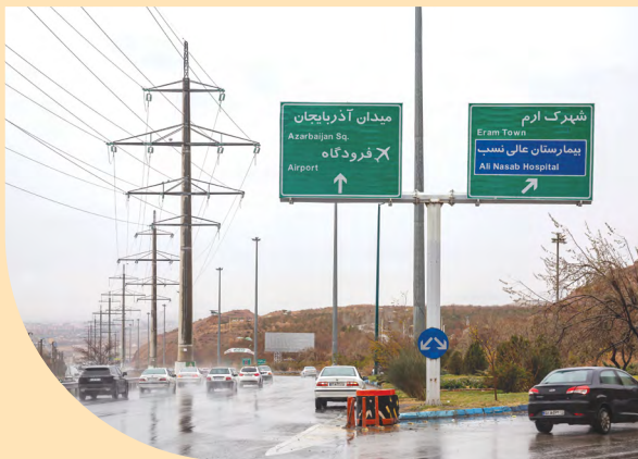
132 kV transmission line on a rainy day along Pasharan Highway in Tabriz, serving as the northern ring road of Tabriz, constructed using Pars Sazeh self-supporting concrete monopole towers.
